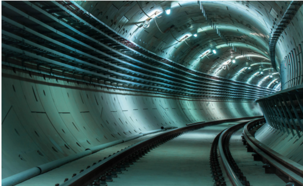
Figure 3 – Tunnel area trackside environment.
