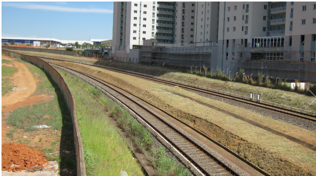
Figure 2 – Open area trackside environment.
